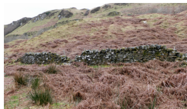
B. Ruined dyke, Isle of Seil
