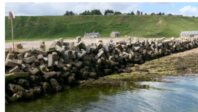
D. Seawall of concrete blocks, Dunbeath
