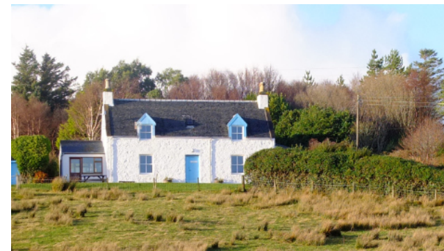
C. House with dormer windows, Loch Ewe
