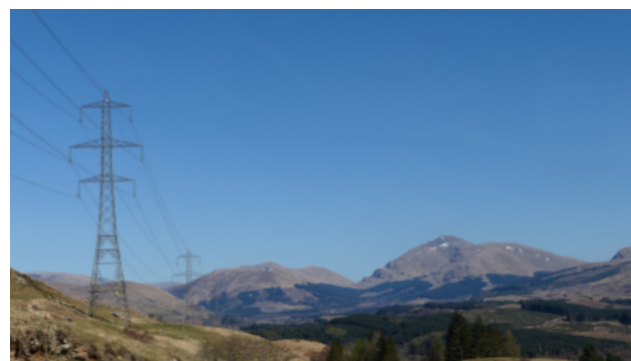
B. Associated electricity pylons, Ben Cruachan
