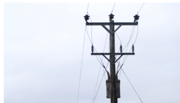
A. Power lines
