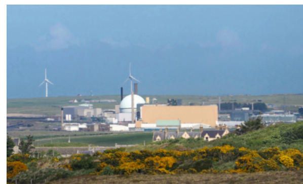
B. Nuclear power station, Dounreay
