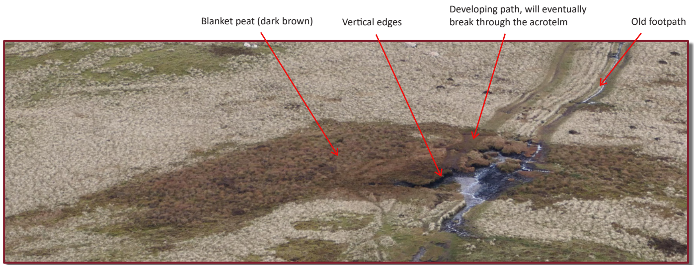
A footpath through a developing area of blanket peat on a hill ridge has broken through the peat, creating a vertical edge. Mechanical damage can be caused by humans, domestic animals, wild animals and vehicles (Pentland Hills)
